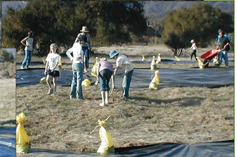
Placing sandbags on top of tarps
